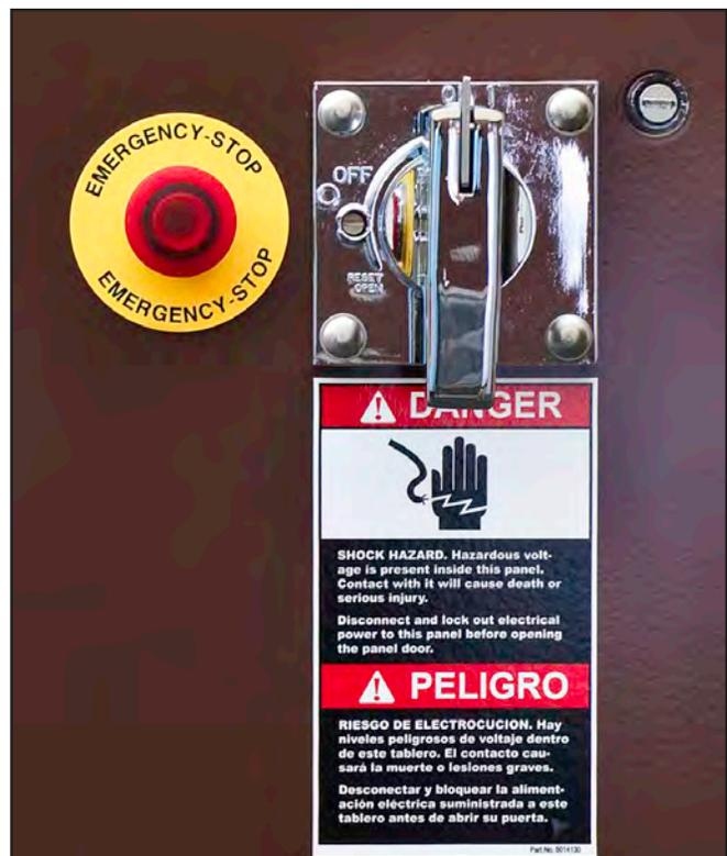
Figure 2. Emergency stop and power disconnect switches.
