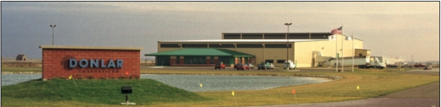
New Donlar manufacturing facility in Peru, Illinois
