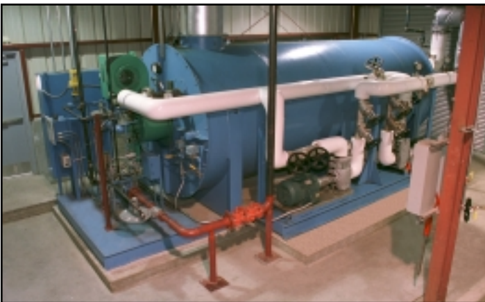
Heatec thermal fluid heater provides process heat for production of polyaspartate polymer
