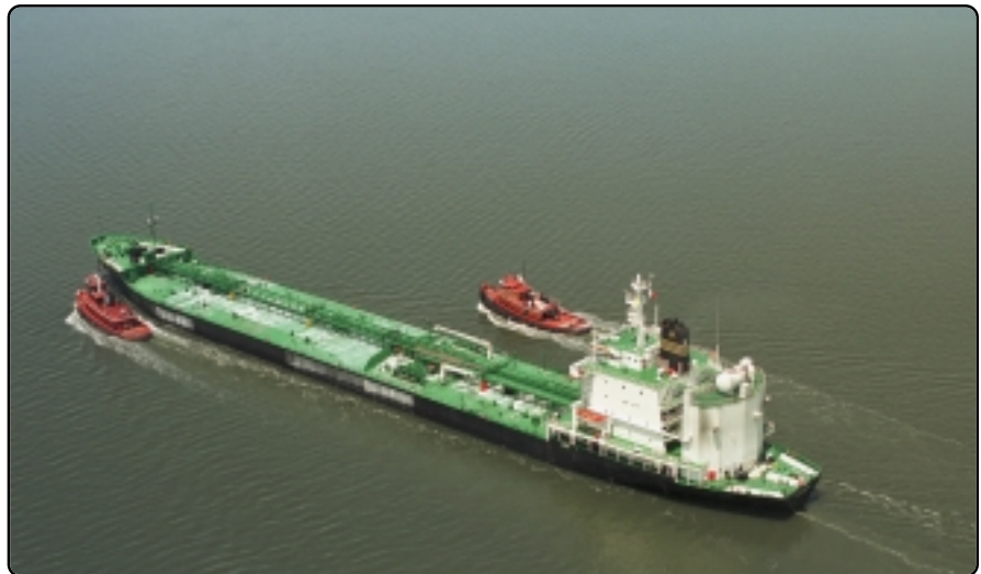
This asphalt tanker has over 22 miles of Heatec piping installed in fourteen compartments. The piping is heated by hot oil supplied by three Heatec helical coil heaters, each capable of providing 15 million Btu/hour.
