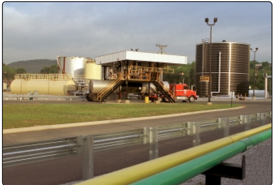
Heatec heating coil modules can be installed in large tanks like the 500,000-gallon asphalt tank shown on the right-hand side of this asphalt terminal picture. A Heatec helical coil heater providing 8-million Btu/hour heats all tanks at this terminal.
