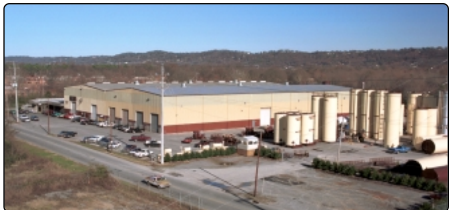
Heatec manufacturing facility in Chattanooga, Tennessee
