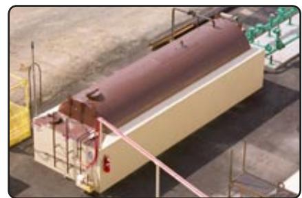
DCT-20 fuel tank with diked construction.
