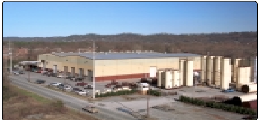
Heatec manufacturing facility in Chattanooga, Tennessee
