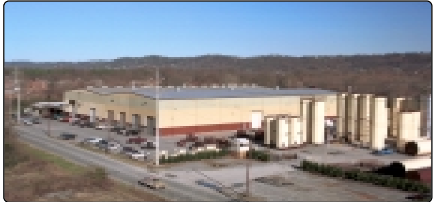
Heatec manufacturing facility in Chattanooga, Tennessee
