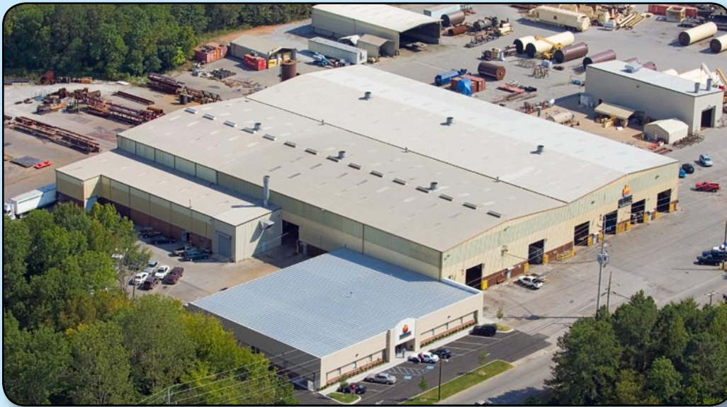
Heatec manufacturing facility and offices in Chattanooga, Tennessee
