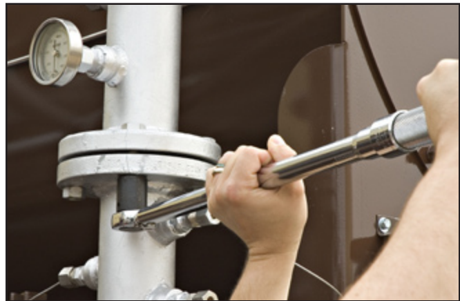
Figure 11. Using a torque wrench to tighten nuts at flanges.
