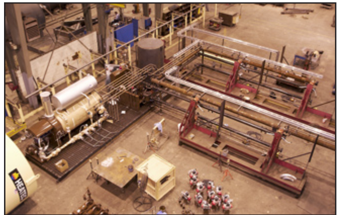
Figure 2. Piping is held by jigs to maintain precise alignment.
