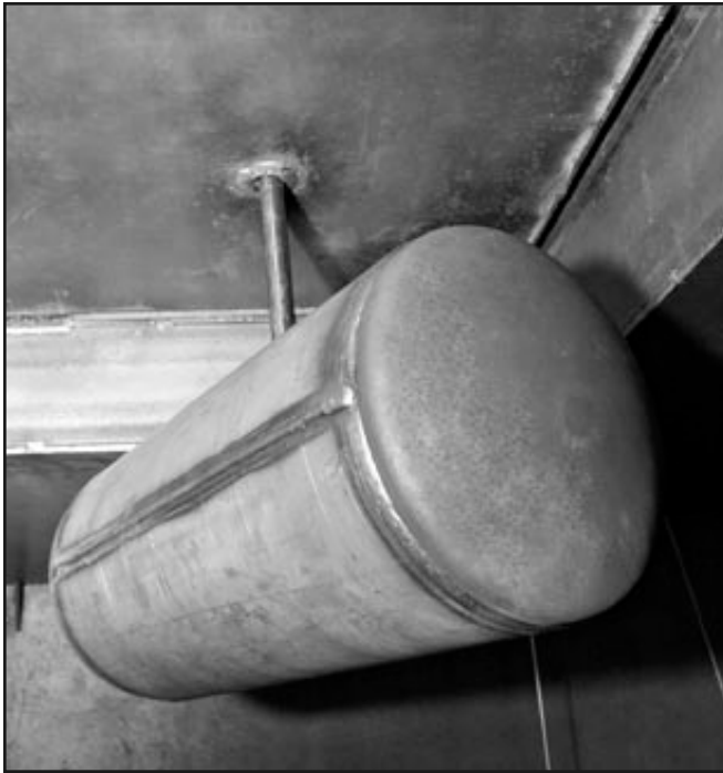
Figure 6. Float for high-level proximity switch.
