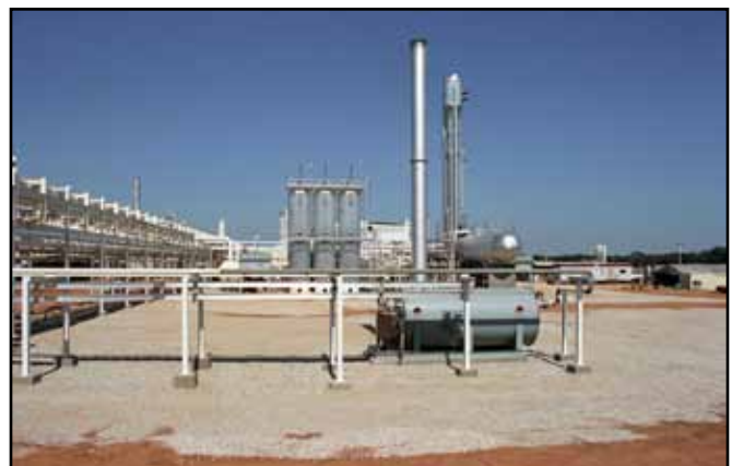
This facility uses two Heatec REGEN heaters to regenerate its gas treatment system. Each heater has an output of 7.1 Btu/hr. One of the REGEN heaters is in the foreground.
