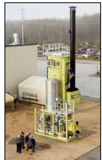
This facility uses two Heatec REGEN heaters to regenerate its gas treatment system. Each heater has an output of 7.1 Btu/hr. One of the REGEN heaters is in the foreground.
