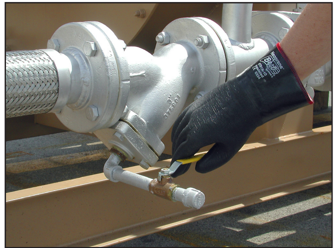
Figure 7. Wear chemical and heat resistant gloves as protection from hot thermal fluid when opening drain valve.
